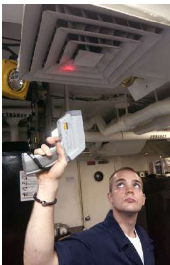
FIGURE 13.5 Fireman Jason Ormand uses a pyrometer to check the temperature of an aircraft carrier's ventilation system. Infrared radiation (whose emission varies with temperature) from the vent is measured and a temperature readout is quickly produced. Infrared measurements are also frequently used as a measure of body temperature. These modern thermometers, placed in the ear canal, are more accurate than alcohol thermometers placed under the tongue or in the armpit. (credit: Lamel J. Hinton/U.S. Navy)
