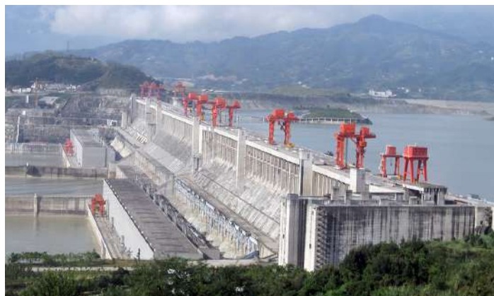
FIGURE 11.4 Three Gorges Dam in central China. When completed in 2008, this became the world's largest hydroelectric plant, generating power equivalent to that generated by 22 average-sized nuclear power plants. The concrete dam is 181 m high and 2.3 km across. The reservoir made by this dam is 660 km long. Over 1 million people were displaced by the creation of the reservoir. (credit: Le Grand Portage)
