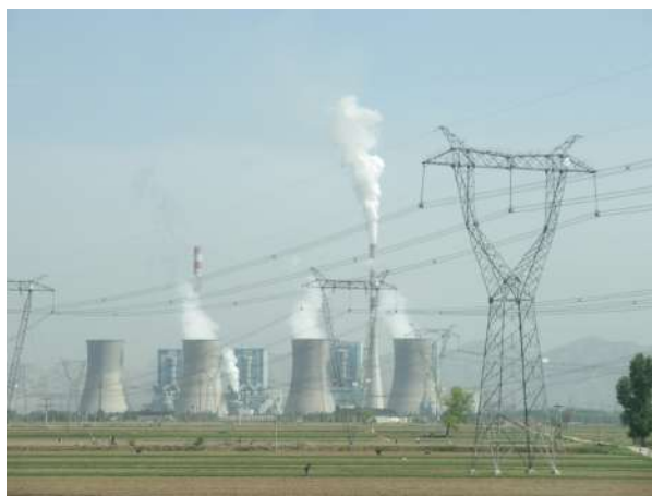
FIGURE 7.22 Tremendous amounts of electric power are generated by coal-fired power plants such as this one in China, but an even larger amount of power goes into heat transfer to the surroundings. The large cooling towers here are needed to transfer heat as rapidly as it is produced. The transfer of heat is not unique to coal plants but is an unavoidable consequence of generating electric power from any fuel—nuclear, coal, oil, natural gas, or the like. (credit: Kleinolive, Wikimedia Commons)
