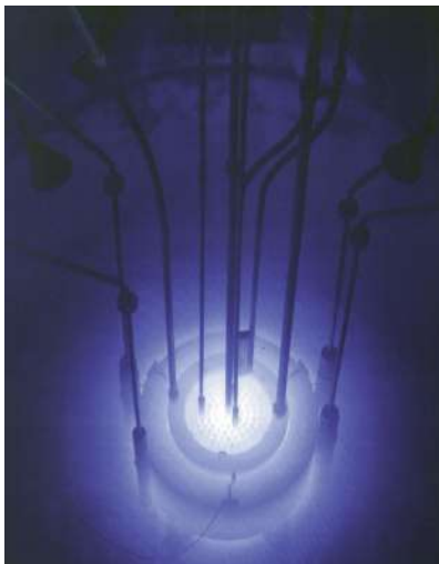
FIGURE 17.19 The blue glow in this research reactor pool is Cerenkov radiation caused by subatomic particles traveling faster than the speed of light in water. (credit: U.S. Nuclear Regulatory Commission)
