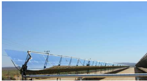
FIGURE 25.42 Parabolic trough collectors are used to generate electricity in southern California. (credit: kjkolb, Wikimedia Commons)
