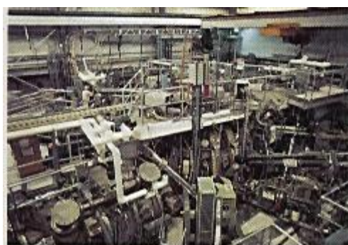
Thermonuclear fusion reactor.
